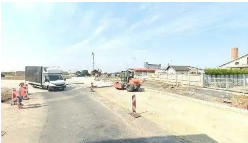
Restaurace cukrovar street view a 360deg
