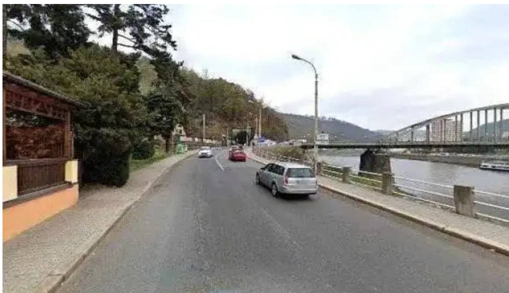
U mostu street view a 360deg
