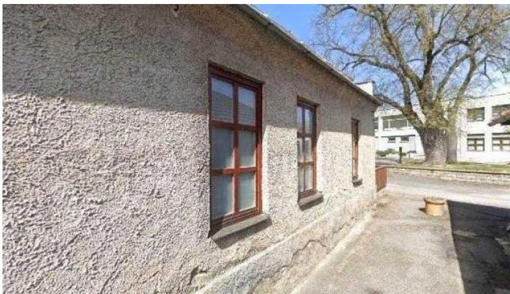
Hospudka na stare radnici street view a 360deg
