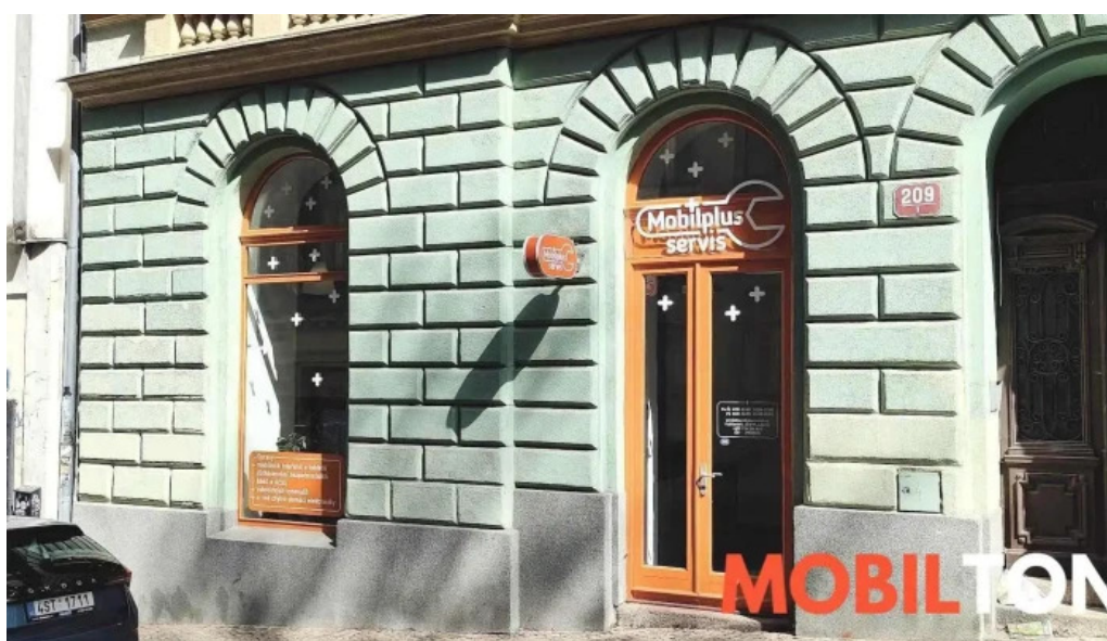
Mobilplus servis exterior
