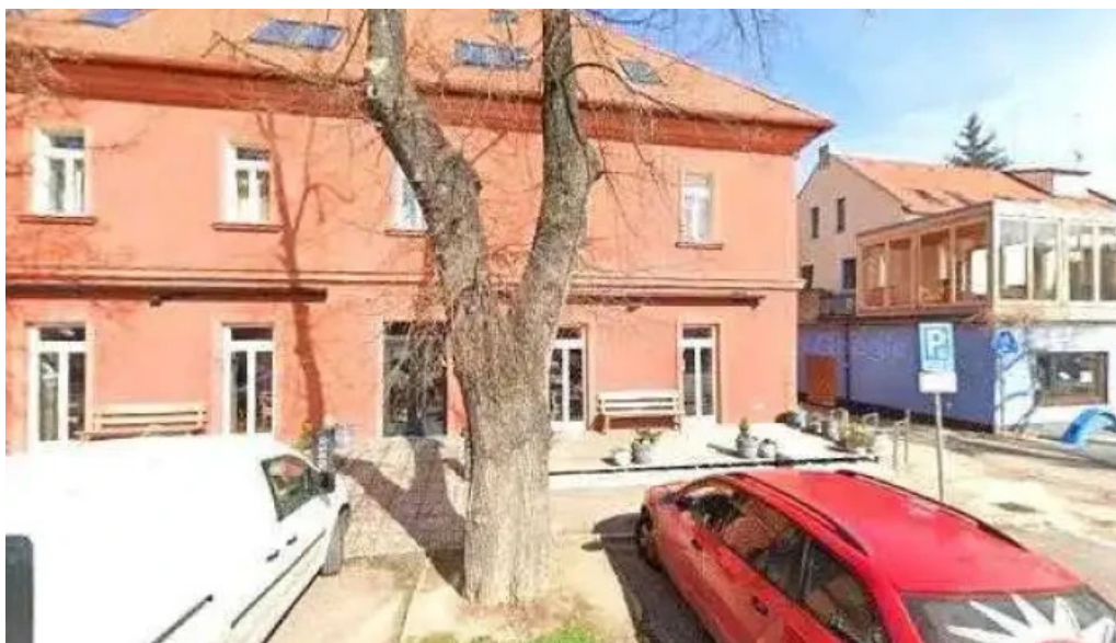
Restaurace corso street view a 360deg
